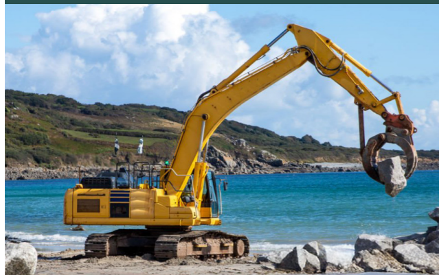
Large Excavator – Repairing Breakwater
