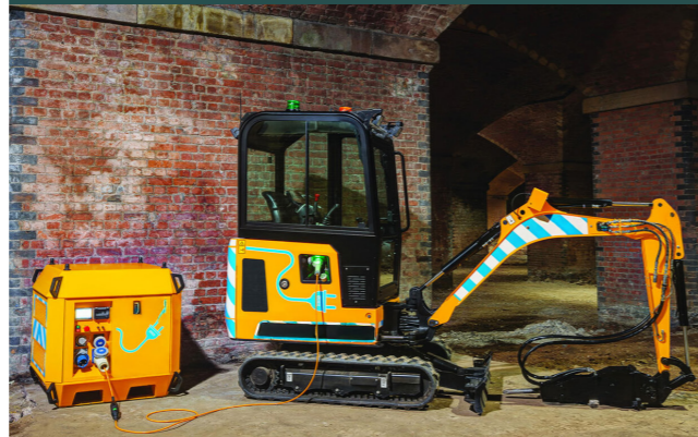
Mini Excavator Working In Basement
